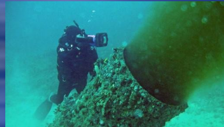
Raw sewage being released directly into the ocean
